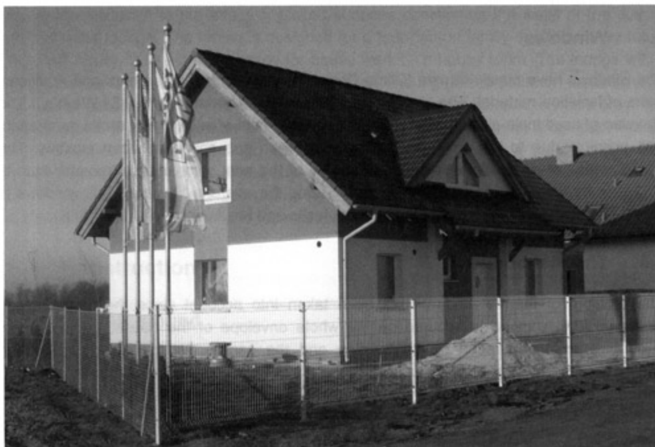
Figure 2: Actual view of north façade of the passive house in Wrocław
