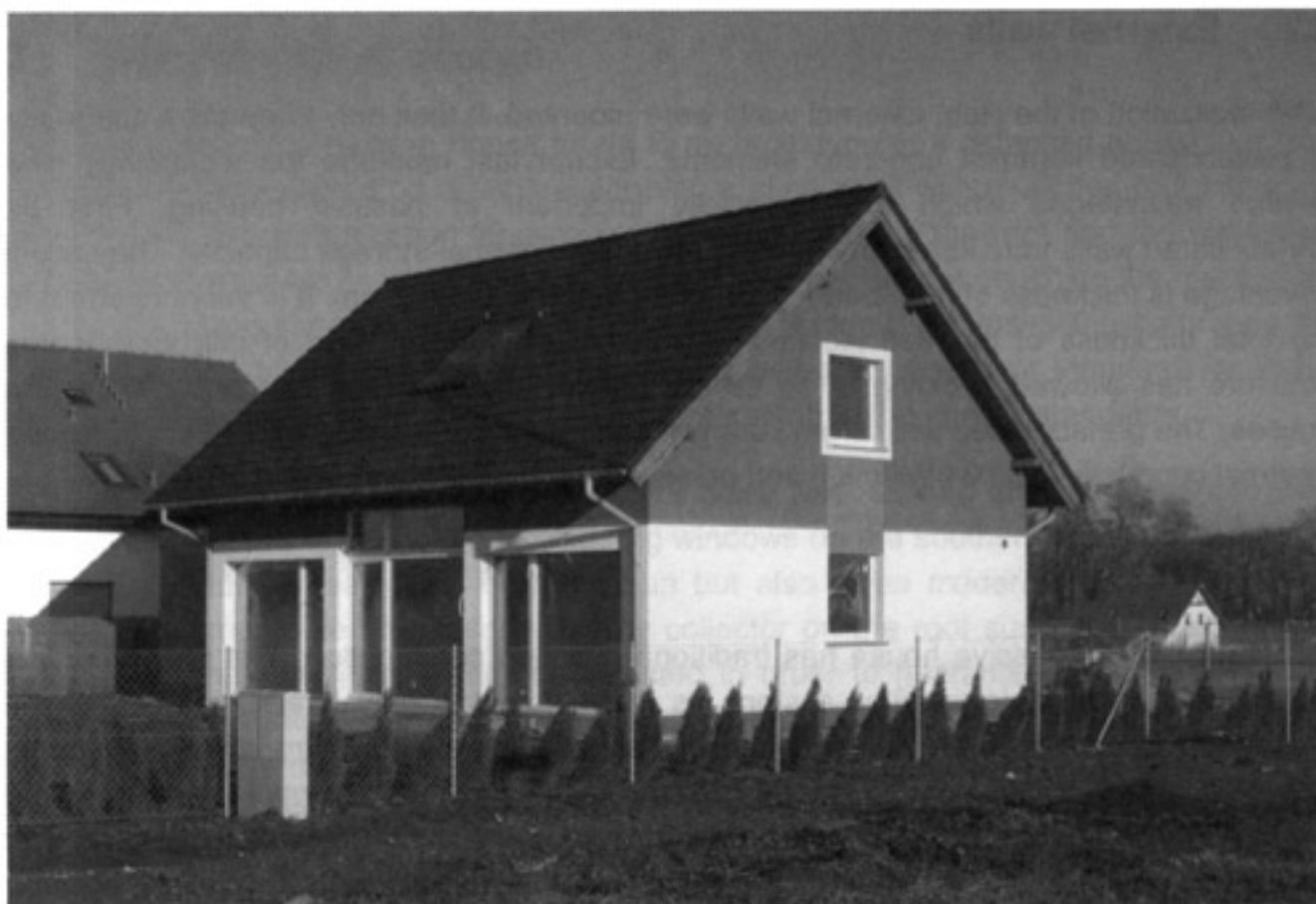
Figure 1: Actual view of south façade of the passive house in Wrocław
