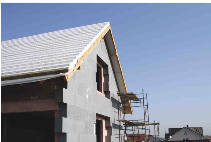
Drawing 5. External dividing structures insulation
