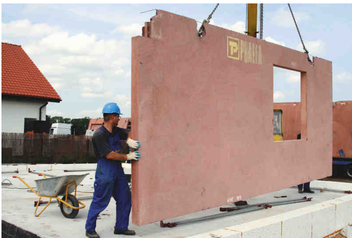
Drawing 4. Installation of the gravelite-concrete prefabricated elements
